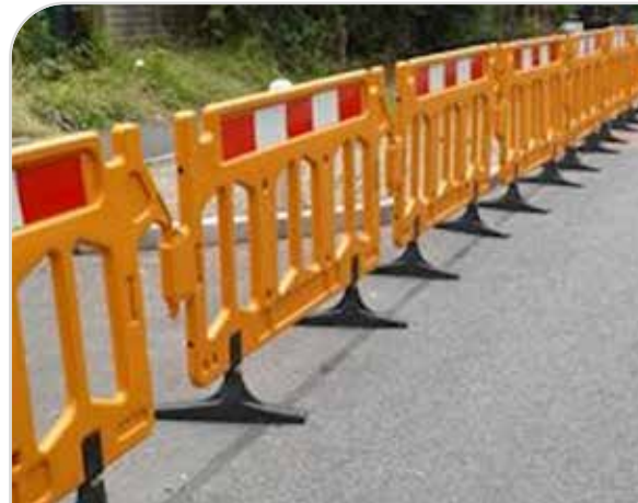
Firmus barriers creating walkway
