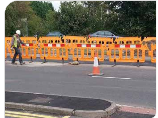
Protection for pedestrian from works
