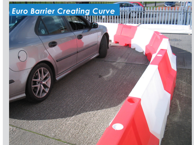
Euro Barriers On Site
